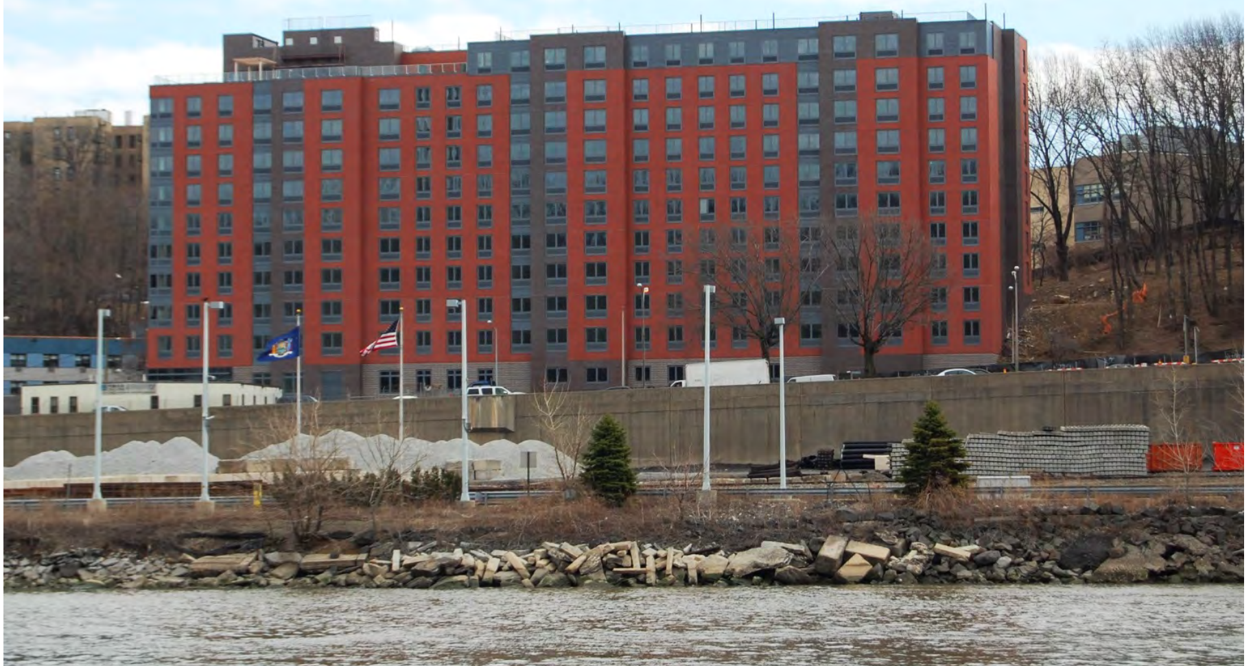
Highbridge Overlook, Bronx
